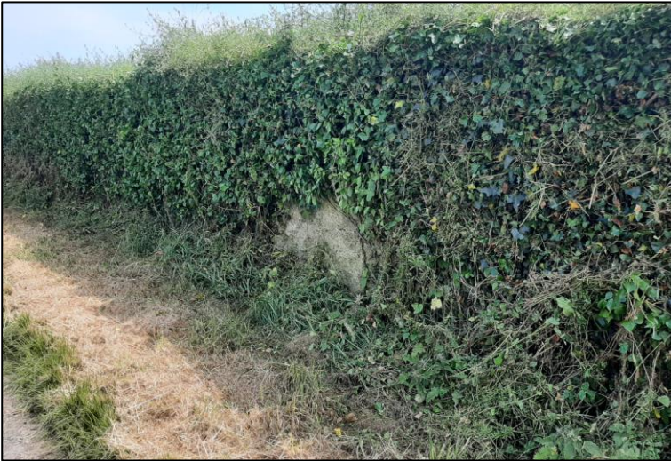
Photo 13.3: Rubblestone Wall Associated with 'Upper Middletown' GDL (DL_15) (Approximate Chainage 36,550)
